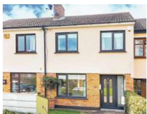
25 Grange Crescent, Dún Laoghaire, Co Dublin
