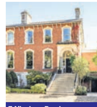
7 Ailesbury Road, Ballsbridge, Dublin 4
