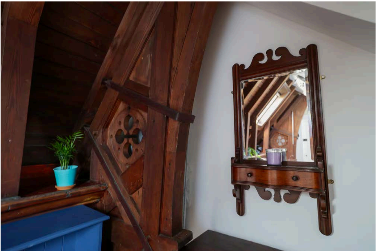
Detailing of rafter joinery. Photograph: Enda O'Dowd
